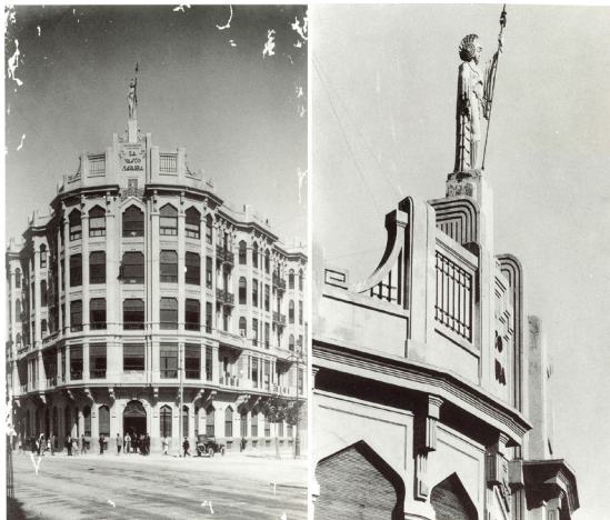
Figure 3. V. Eusa. Vasco-Navarra building.
