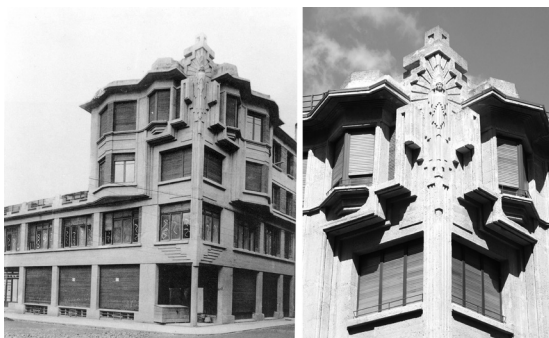
Figure 4. V. Eusa. Residential building in García Castañón street.
